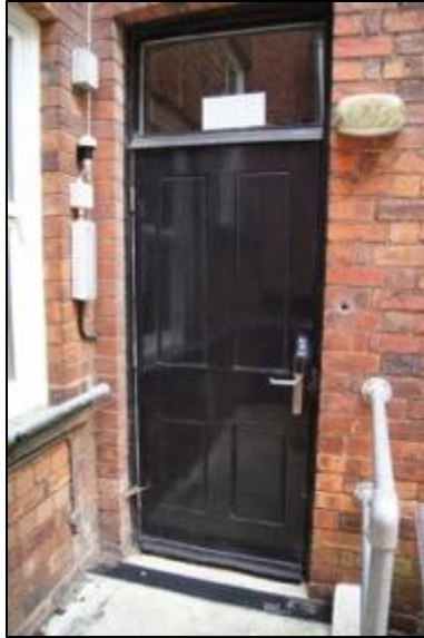
This photograph shows the supplementary accessible door.
